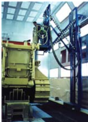
Paint/Preparation Booth: 3-Axis Lift System for painting large construction equipment
